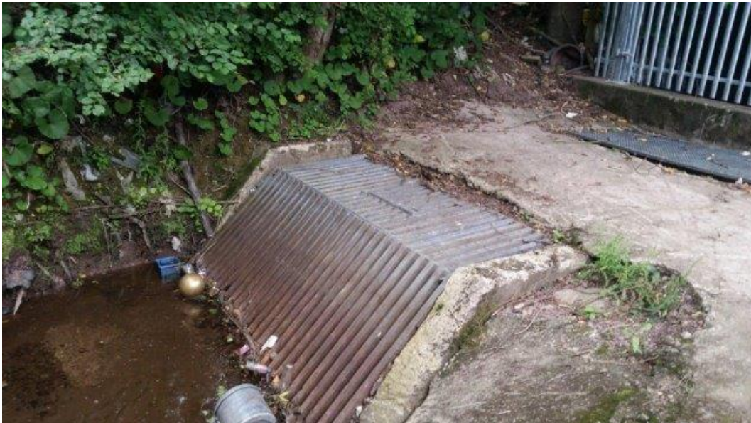
Figure 3.13: Existing trash screen at Lehenaghmore Industrial Estate
