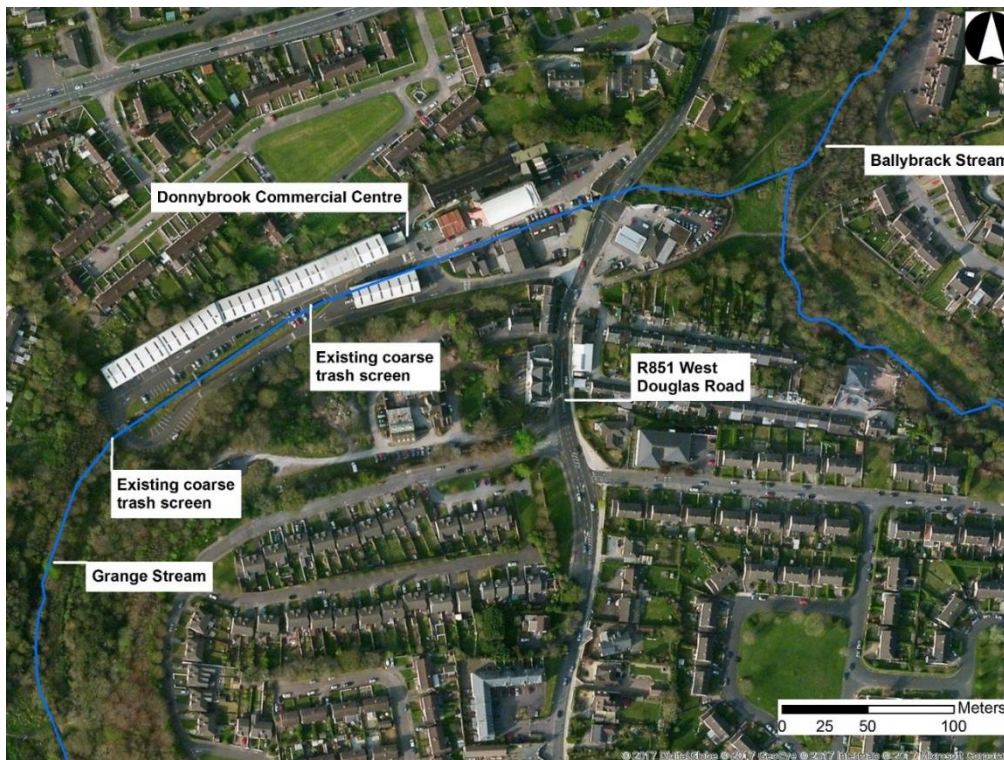
Figure 3.8: Donnybrook Commercial Centre (Area 3) showing the Grange Stream.
