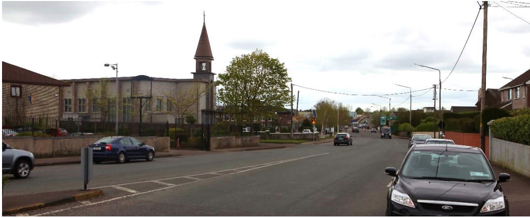
Figure 3.12: View of Togher Road (looking north), including the Church of the Way of the Cross. The proposed flood defence scheme culvert runs under and along the western pavement of Togher Road.
